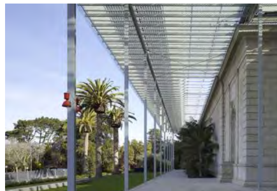
PHOTOVOLTAIC COVERED WALKWAY GALLERY OF CALIFORNIA ACADEMY OF SCIENCES BY RENZO PIANO ARCHITECTS
