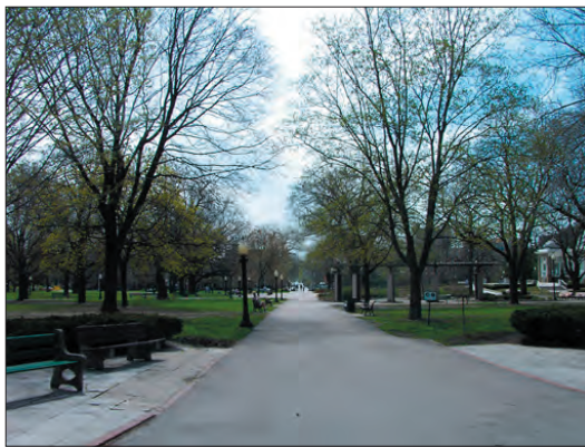
The use of asphalt as a paving material along the axial path is inappropriate. Restoration should include the concrete surface with the forced perspective as seen in historic photographs. (Photo credit: D833-jjs 0652)
