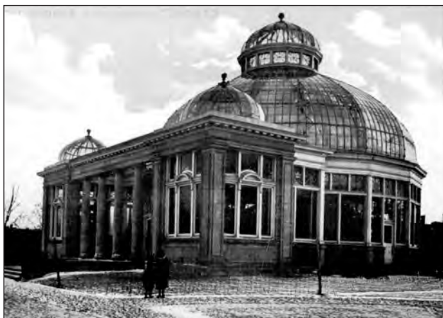
The Palm House in late 1910 or early 1911. Plant material installed indoors but hoarding still up outside. (Photo credit: TRL T34932)
